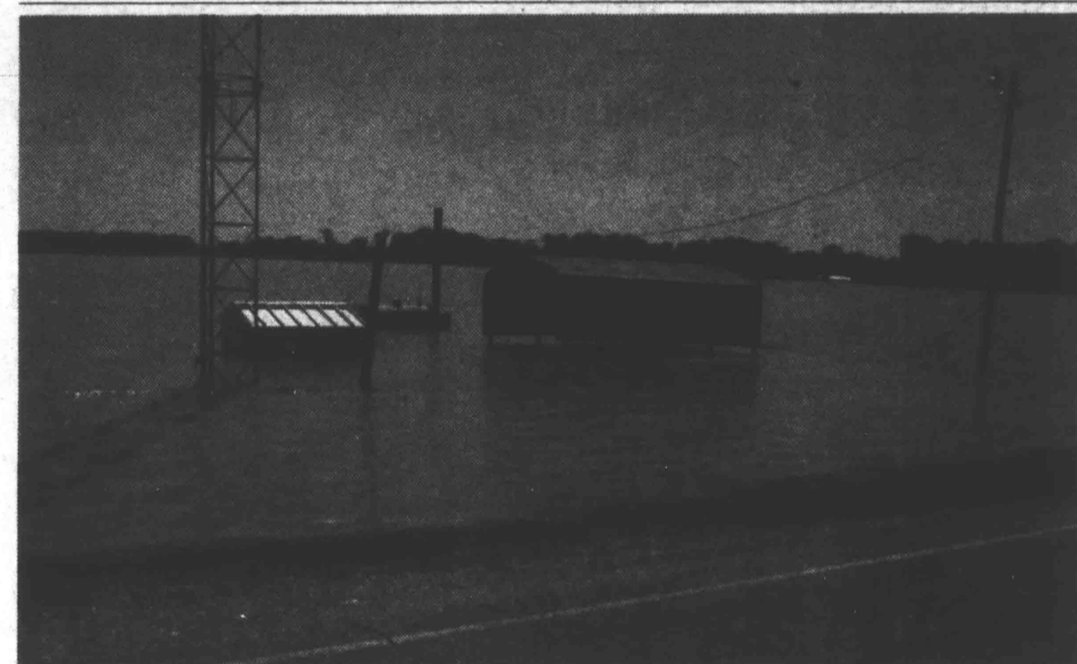
GAS SUBSTATION, ON ESPY PARK RD., NEAR HALLS
